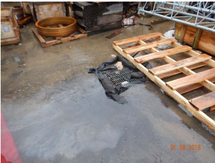
Photo 3. Drop inlet located near the southwest corner of the Facility. Note the sheen flowing into the drop inlet.
