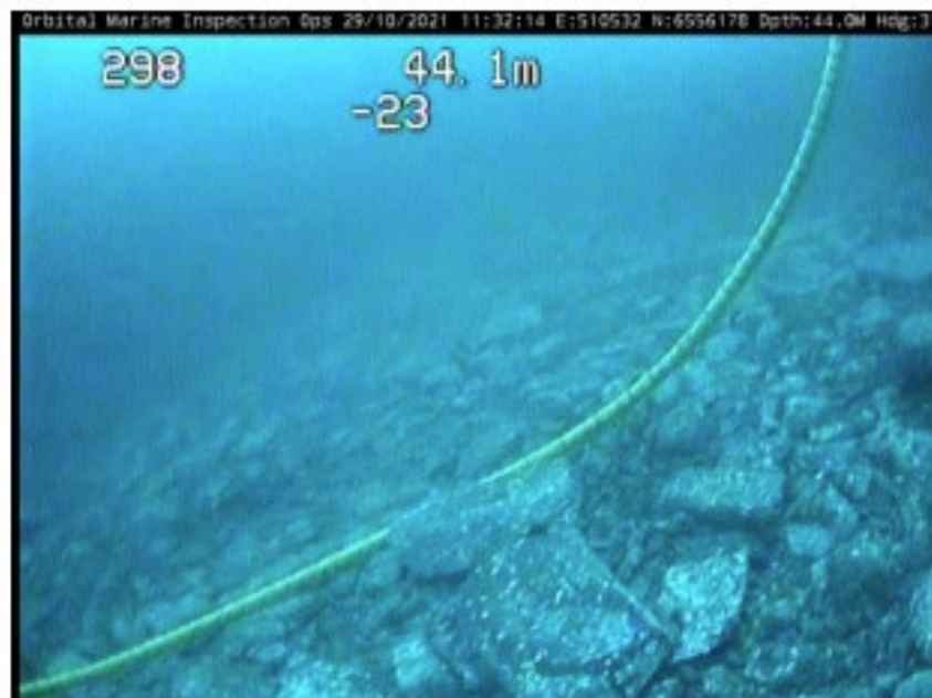
Figure 72. Typical Orbital O2-X Subsea Cable Slack
