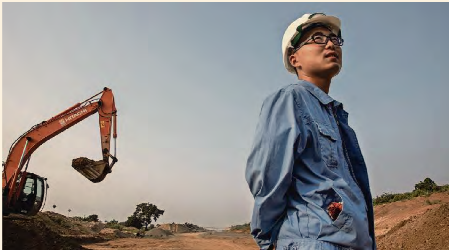
Foreign help: a Chinese site engineer works on an extension of the Southern Expressway in Sri Lanka in 2018
