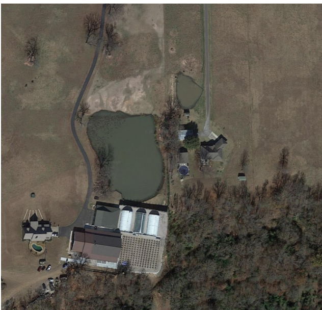
Aerial view of the Grants' property and Bacon's property following the construction of Flying Bud.
