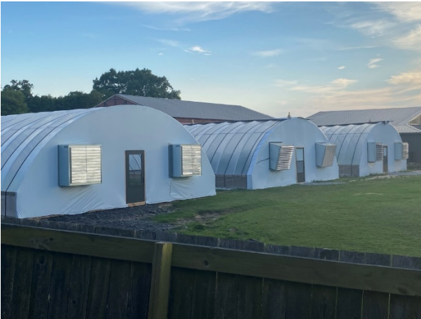
View of the illegal marijuana operation's completed grow houses and industrial fans from the Grants' property.
