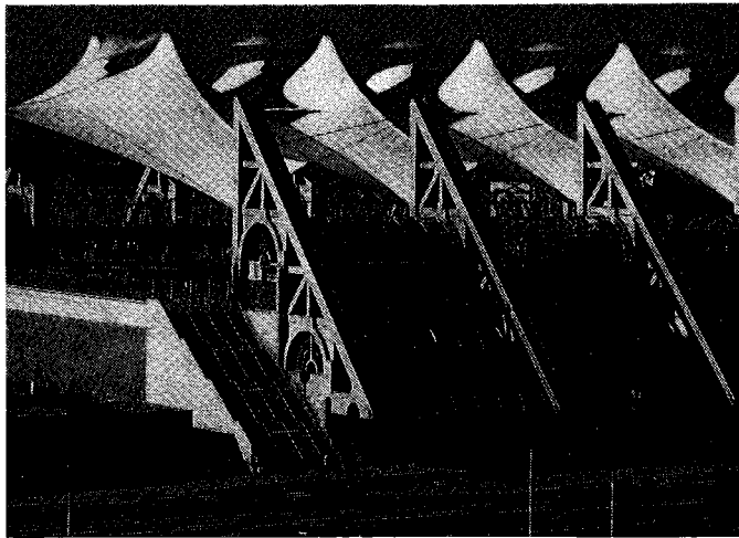
FIGURE 6.13 San Diego Convention Center, San Diego, California (courtesy of Birdair, Inc.).
