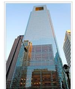
The Comcast Center in Philadelphia, headquarters of Comcast
